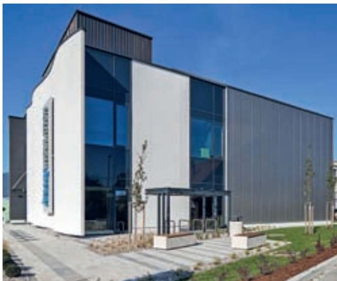
Knauf Insulation Experience Center, Škofja Loka
